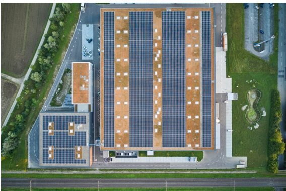
The solar power plants on the roofs of the Forster Campus generate up to 15 MWp of electricity per year and provide sustainable energy for production and building operations. Photo: © leader.ch
