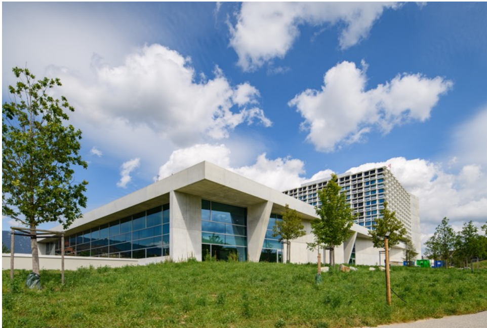
Highly efficient heat protection was important for the glazing of the base structure, which is achieved with triple insulating glass from Glas Trösch. Photo: Glas Trösch
