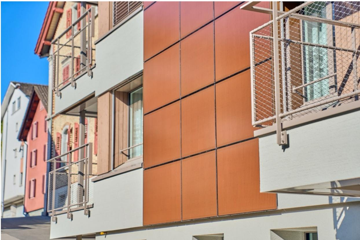
Only upon closer inspection do the PV modules reveal themselves. The absence of frames enhances the seamless aesthetic. Photo: 3S Swiss Solar Solutions AG
