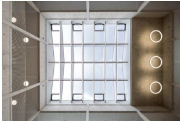
An innovative sun protection grid ensures optimal, glare-free use of daylight.
